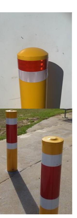
These bollards have all been impacted by a vehicle but shown here are bollards installed using the Impact Recovery System. The red one has been hit several times (once by a large truck) but although the footings are scuffed, they, and the bollard remain in pristine condition (has been repainted)
